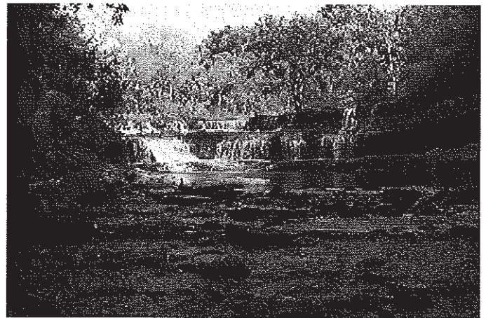
Rock Creek Spillway at Fort Scott
