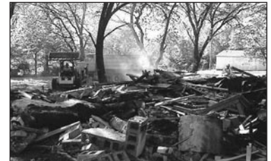
Onaga PRIDE volunteers demolish an old house.
